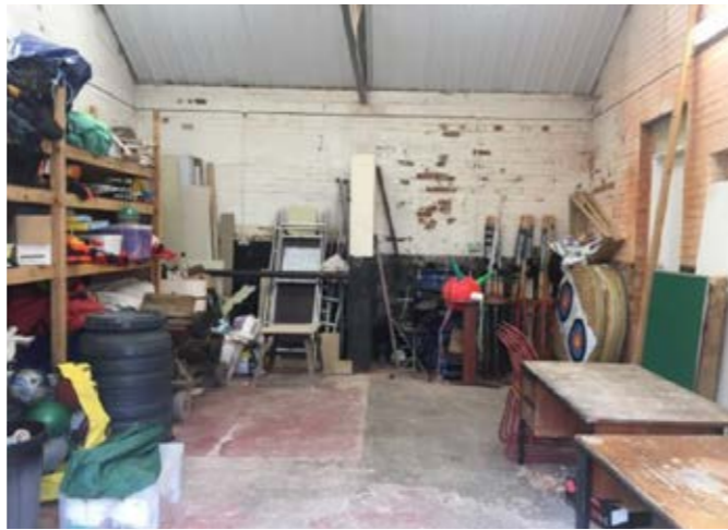
Above Storage room pre-conversion
